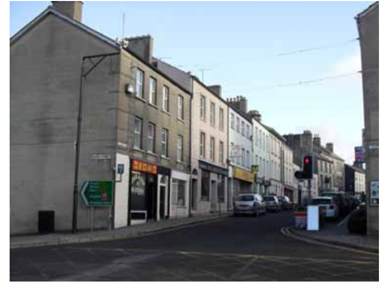
Shop front improvement schemes are often very successful in raising the profile of an area. This is especially true where there is an historic town core with many fine buildings that have not been as well maintained as they might have been.
