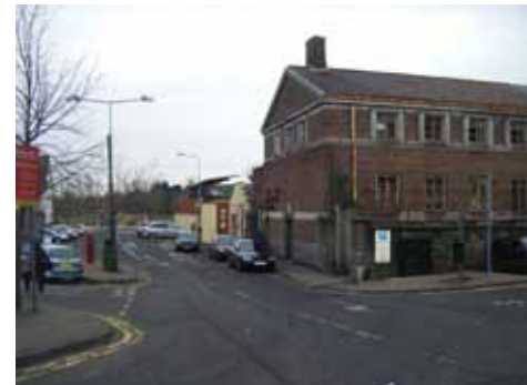
There are a number of commercial activities in key locations which might be relocated, thus freeing up land for development
