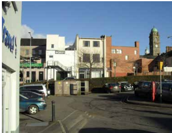
Enniskillen tends to face 'inwards' towards the main thoroughfare, but there are a number of locations where rear building facades and back court areas can become part of the overall town centre experience. Alleyways leading to small courtyards, with shops, cafes and restaurants can add considerable charm to the town centre.
