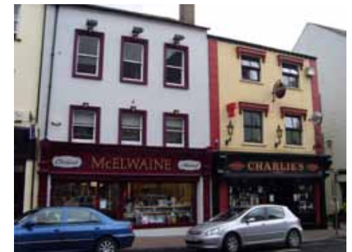
Existing building frontage improvements in Enniskillen
