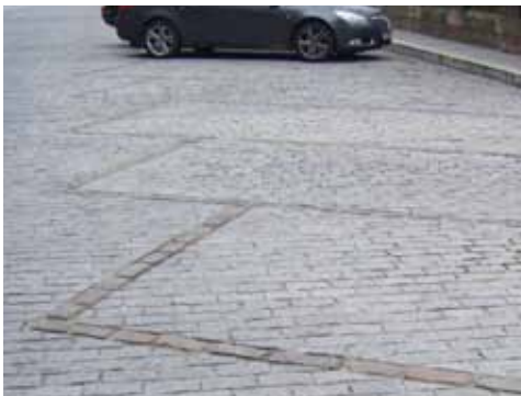
Parking bays marked out with granite setts
