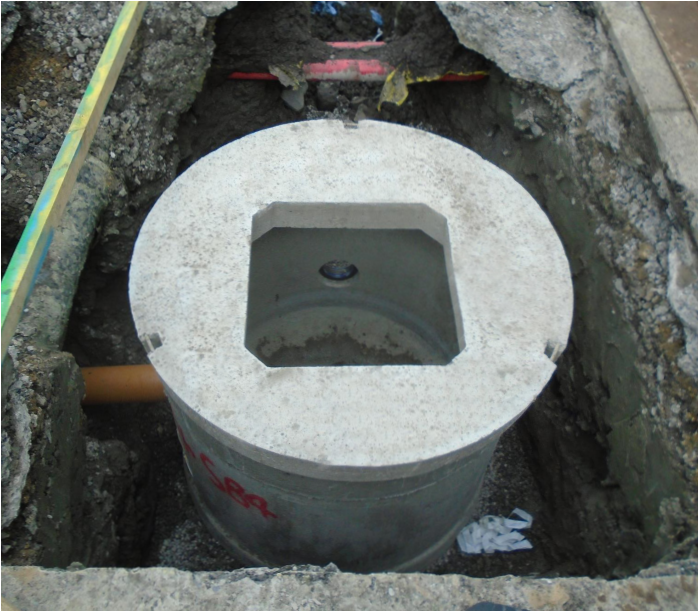
FP McCann Precast Manhole Installation
