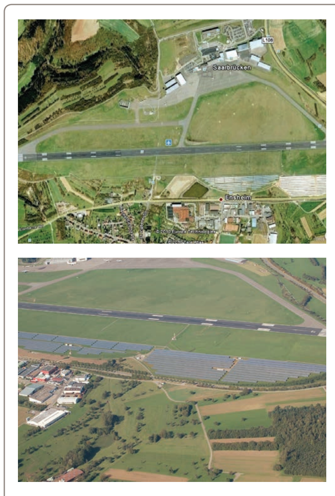
Figure 24 East Langford 5MW solar farm, Cornwall. Image courtesy of Low Carbon Solar
