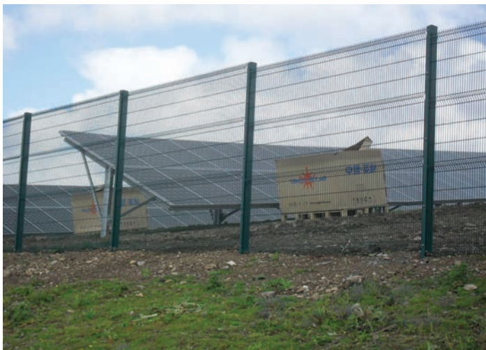
Figure 11 Close welded mesh panel fencing, as shown here at the Wheal Jane solar farm, generally has a low landscape / visual impact while also being versatile and providing a good level of site security.
