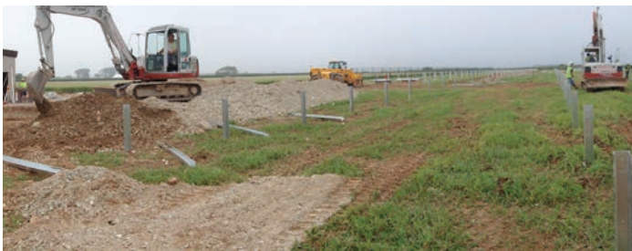
Figure 2 Development of the 5MW Trenouth solar farm, Cornwall. Images courtesy of Inazin.
