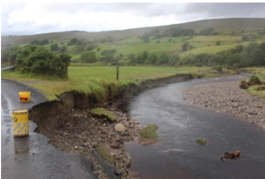
Flood Damage – Davagh Road [Coneyglen] Aug 2017
