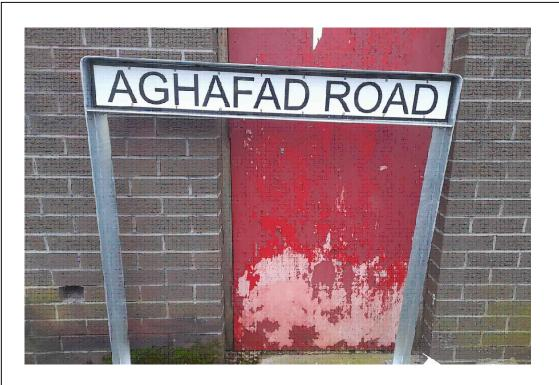
Sign Plate to be riveted to the aluminum rails at 75mm , centres top and bottom
