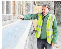
CHECK... Kevin Boggs working on the original sash windows.
