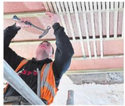
LOOKING UP... Working on repairing the ceiling.
